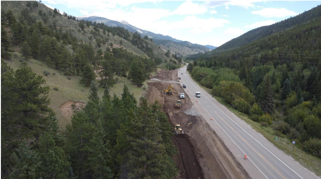
Grading and excavation on the west side of CO 285 near Grant.
